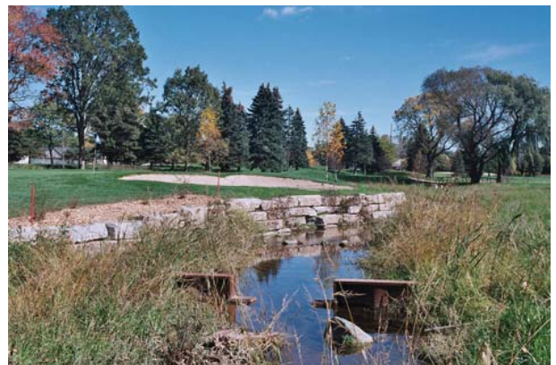
Sylvan Glen Golf Course Weir and Streambank Stabilization
