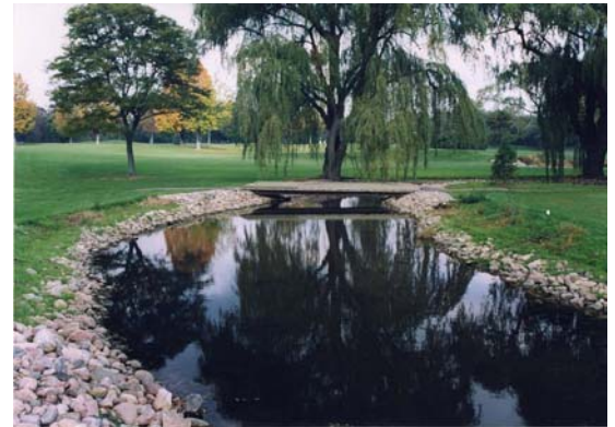
Springdale Golf Course Streambank Stabilization
