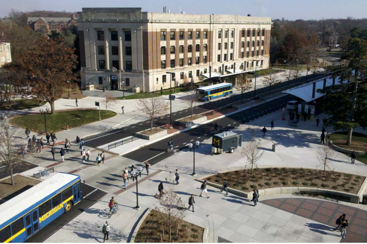
Top left: University of Michigan Central Campus Transit Center
